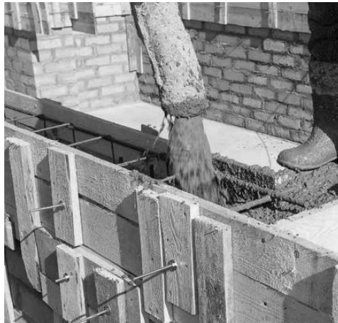
Figure 9. Concrete Casting Process for Lintel Beams
