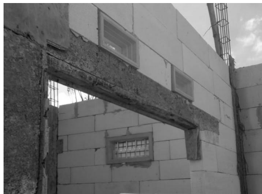
Figure 10. Finished Lintel Beam
