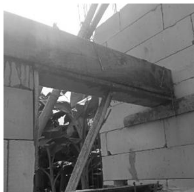
Figure 8. Concrete Lintel Beam Formwork
